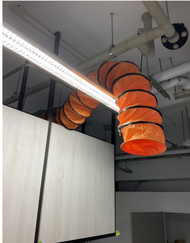
Figure 12: Photo of the additional air duct installation.
